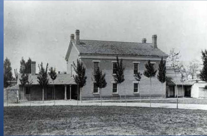
Temporary structure used during the construction of the Salt Lake Temple--1855
