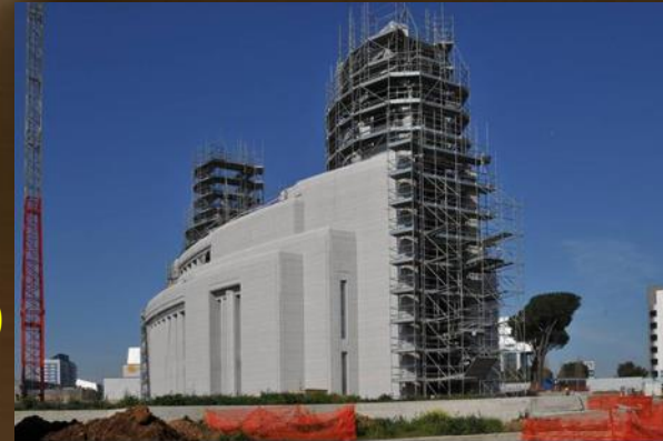
Construction of Rome, Italy Temple
